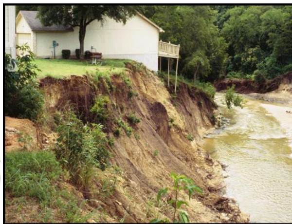
Figure 2: Picture of Stream Erosion in Texas
